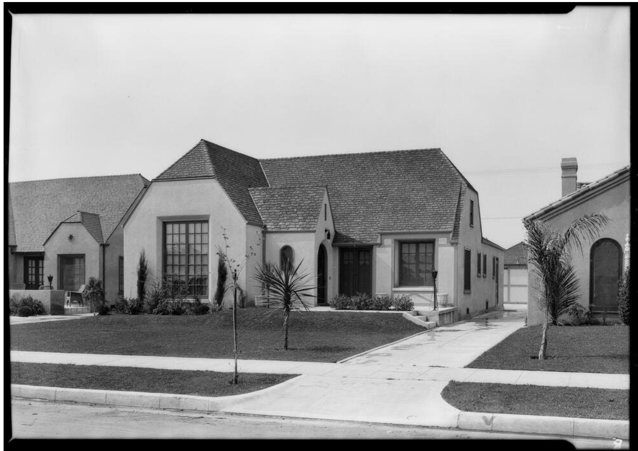
Figure 1 Single family house at 117 N. Citrus Avenue, 1926, photographer: Dick Whittington; Source: USC digital library, house demolished 2016
